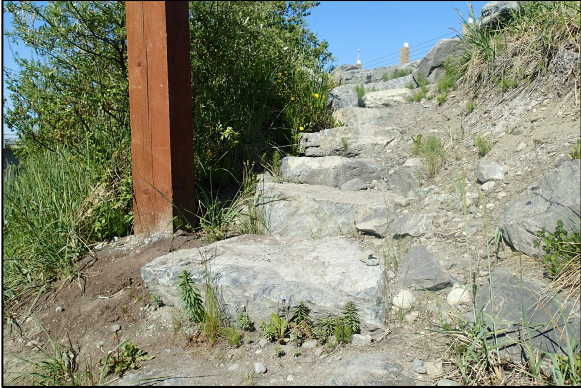
Figure 8. An example of a set of stone steps installed during the Phase II improvements; the wooden post supports signage indicating the location of the steps (May 2015).
