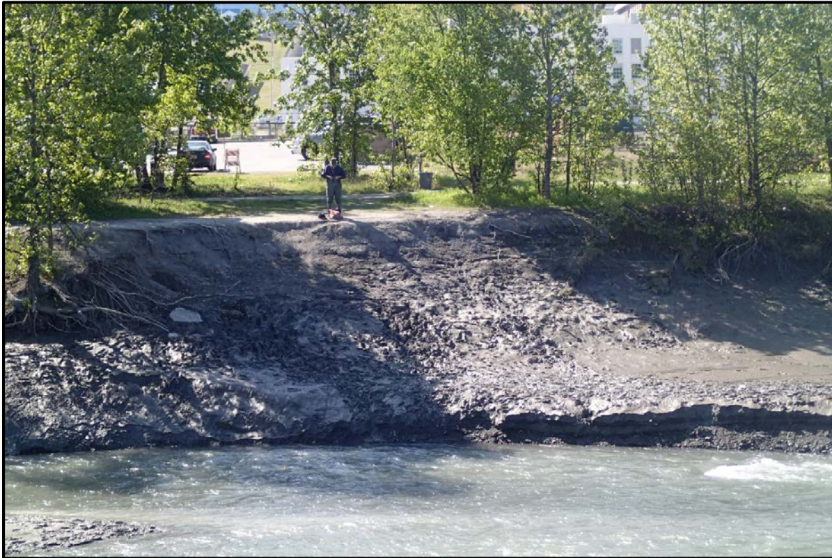
Figure 7. A portion of stream bank along the South Bank Trail showing signs of heavy foot traffic. The man in the photograph is standing at the location of the proposed Stream Bank Trail overlook as shown on figure 6, and a set of stone steps is proposed for the stream bank below him (May 2015).
