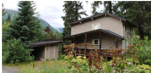
Figure 99. 2911 Alyeska Highway, view to the northwest.
