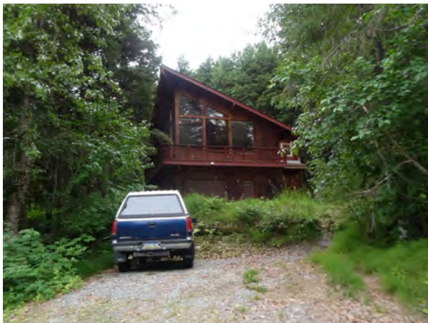
Figure 40. 153 Juniper Drive, view to the south.
