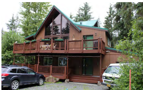
Figure 125. 138 Northland Road, view to the northwest.
