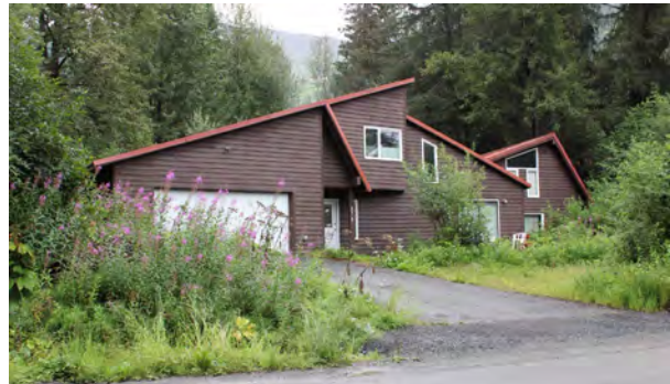
Figure 94. 570 Alyeska View Avenue, view to the east.
