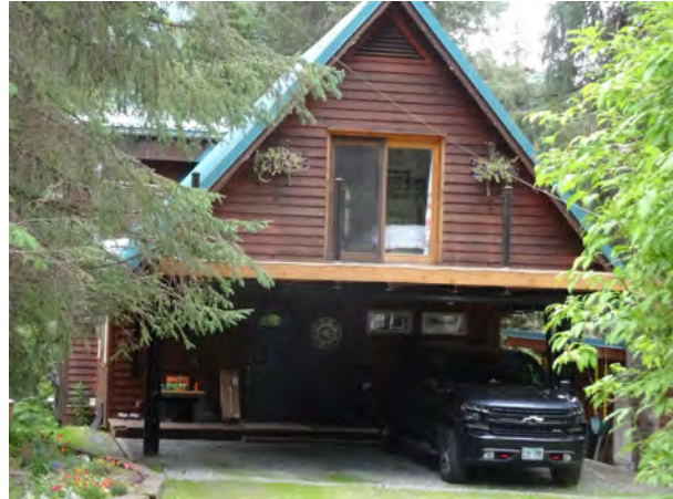
Figure 43. 148 Beirne Street, view to the southeast.
