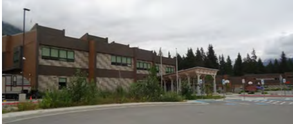
Figure 78. Girdwood Elementary School, view to the north.
