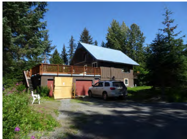
Figure 167. 318 Davos Road, view to the north.
