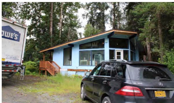
Figure 124. 110 Northland Road, view to the west.
