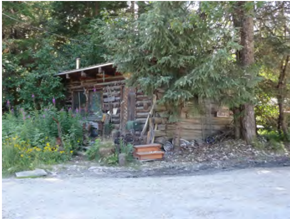
Figure 75. 373 Crow Creek Road, view to the south.
