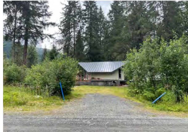
Figure 144. 305 Brighton Road, view to the south.
