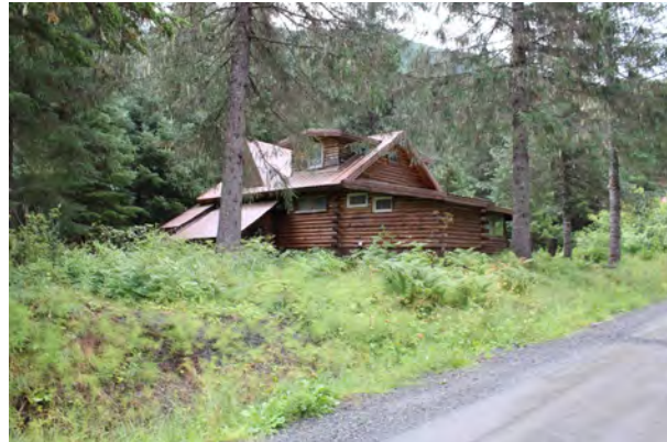
Figure 117. 566 Alpine Meadows Avenue, view to the east.
