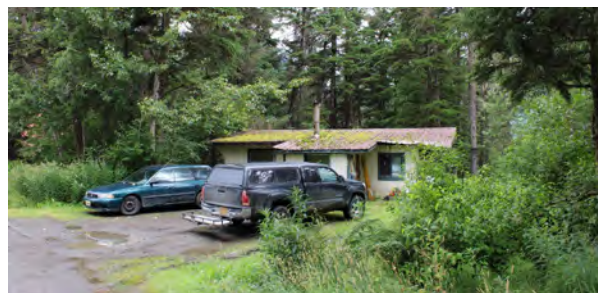
Figure 126. 166 Northland Road, view to the northwest.
