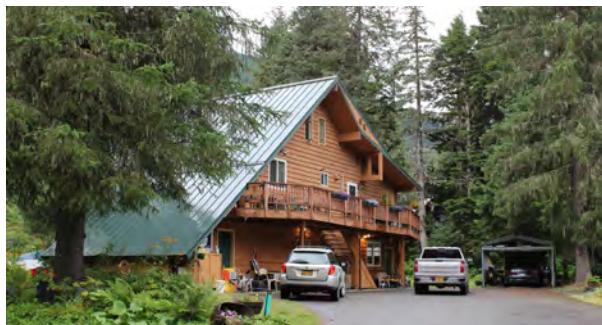
Figure 130. 163 Cortina Road, view to the south.
