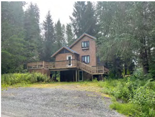
Figure 143. 273 Brighton Road, view to the south.
