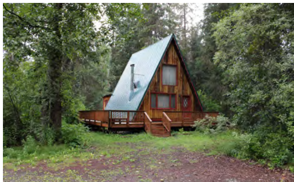
Figure 10. A-Frame residence located at 220 Cortina Road in Girdwood, Alaska.
