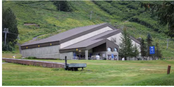
Figure 146. 104 Arlberg Avenue, view to the southeast.
