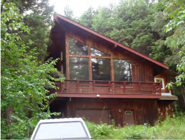
Figure 13. Prow Front style residence at 153 Juniper Drive in Girdwood, Alaska.
