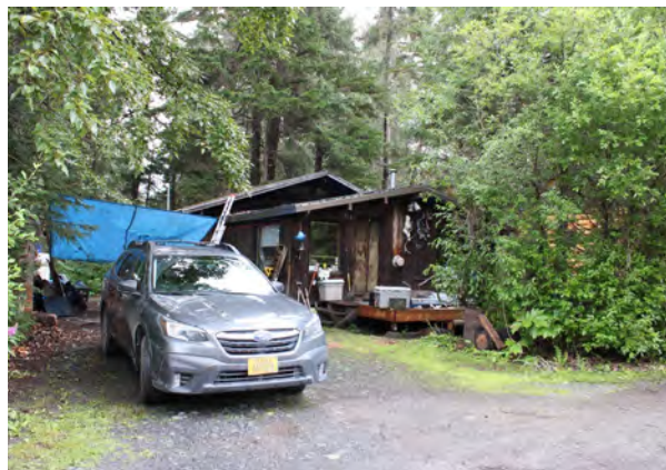
Figure 109. 160 Innsbruck Road, view to the north.
