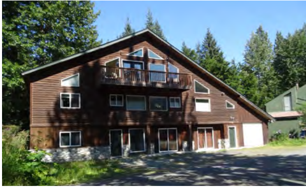
Figure 165. 267 Donner Drive, view to the west.
