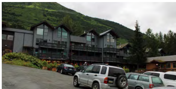
Figure 179. 194 Olympic Mountain Loop, view to the east.
