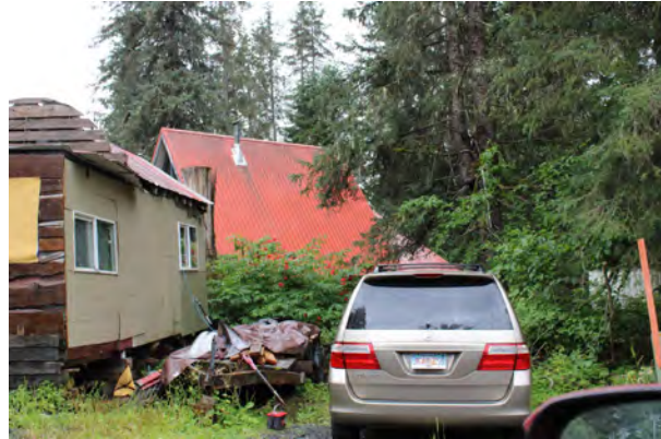
Figure 105. 225 Garmisch Road, view to the south.
