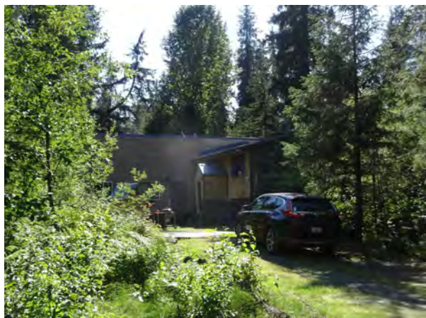
Figure 157. 143 Aspen Mountain Road, view to the southwest.
