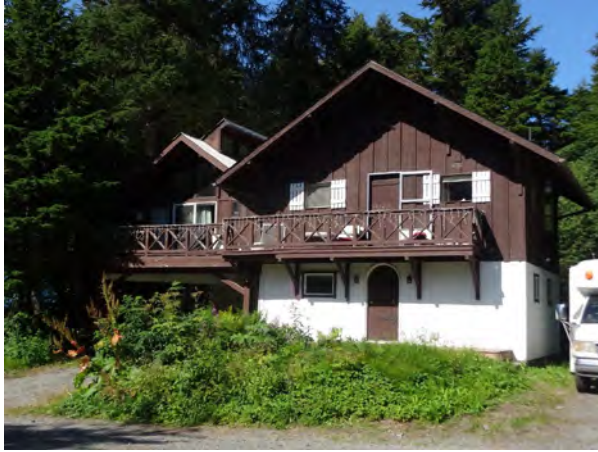
Figure 11. Swiss Chalet style residence located at 214 Brighton in Girdwood, Alaska.
