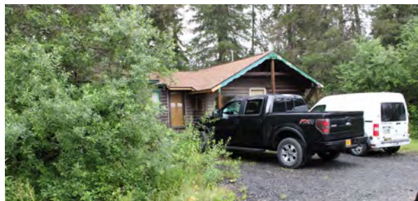
Figure 133. 257 Cortina Road, view to the south.
