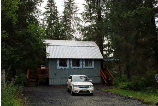
Figure 110. 119 Kitzbuhel Road, view to the south.
