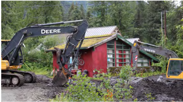
Figure 86. 916 Alpine Meadows Avenue, view to the east.
