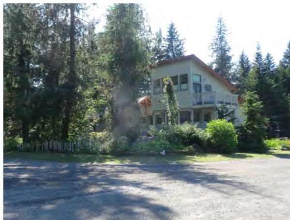
Figure 156. 847 Alyeska View Avenue, view to the southwest.
