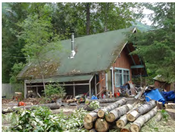
Figure 54. 222 Hottentot Mine Road, view to the northwest.
