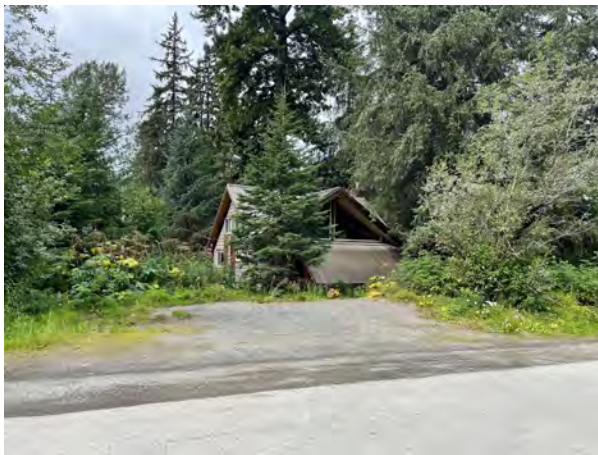
Figure 93. 569 Alyeska View Avenue, view to the northwest.
