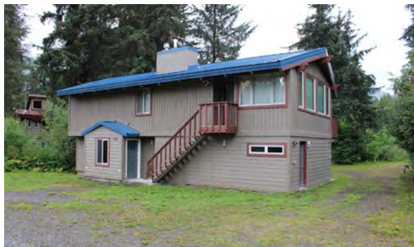
Figure 108. 102 Innsbruck Road, view to the north.
