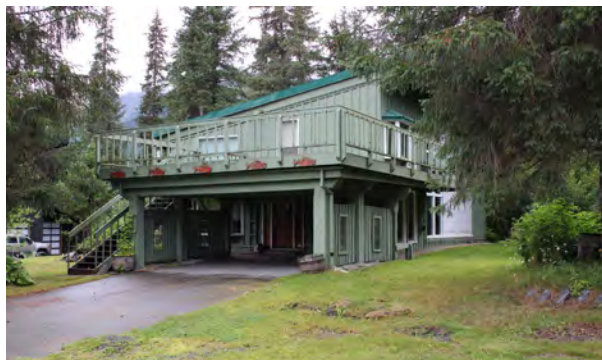
Figure 140. 242 Davos Road, view to the northeast.
