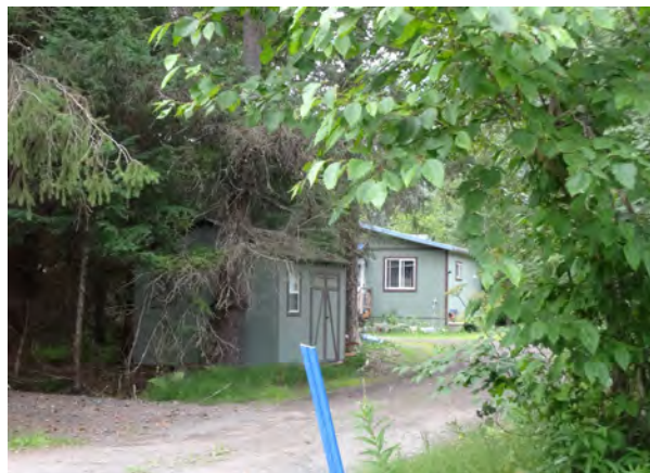
Figure 49. 355 Sproat Road, view to the southwest.
