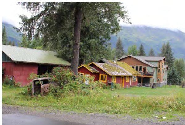
Figure 135. 110 Davos Road, view to the northwest.
