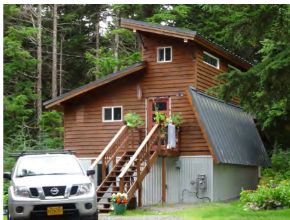
Figure 37. 157 Doran Lane, view to the south.
