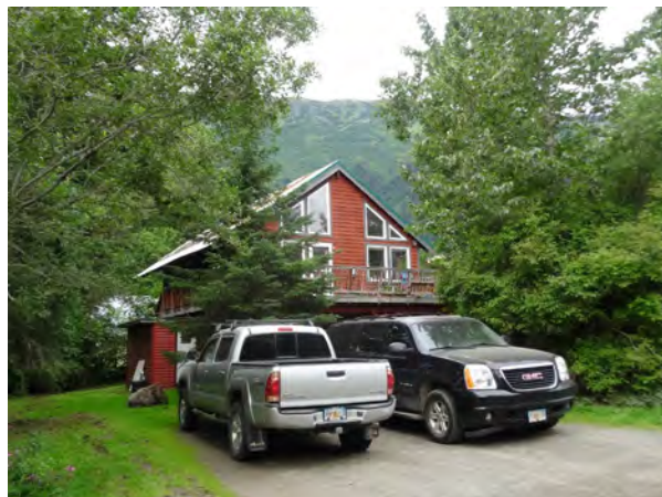
Figure 48. 225 Sproat Road, view to the northwest.
