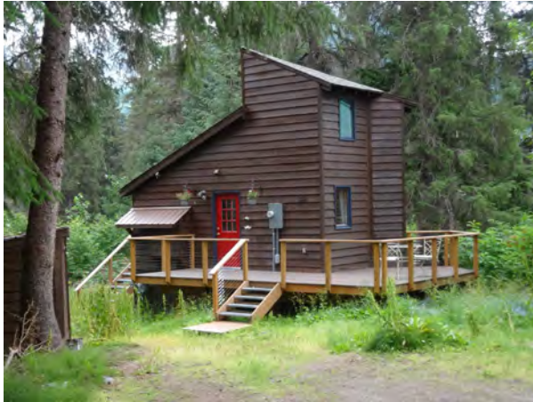
Figure 42. 144 Beirne Street, view to the southeast.
