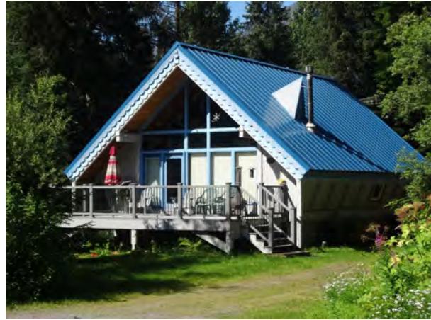
Figure 12. Modern Chalet style residence at 228 Brighton Road in Girdwood, Alaska. This is an excellent unaltered example of the Haida Hide Home.
