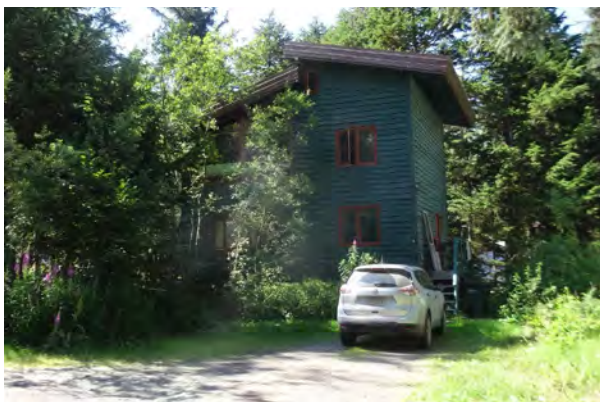
Figure 163. 191 Donner Drive, view to the west.
