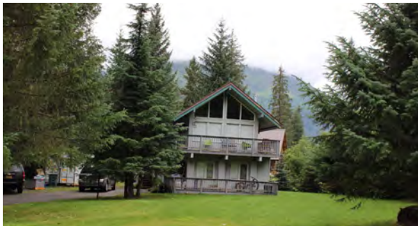
Figure 137. 144 Davos Road, view to the north.
