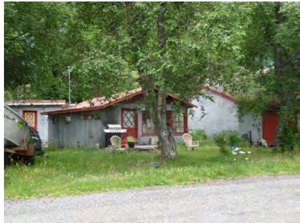
Figure 82. 237 Main Street, view to the west.
