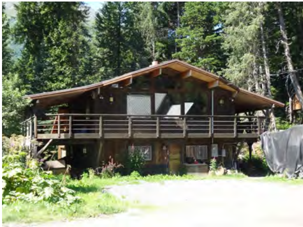
Figure 160. 151 Donner Drive, view to the west.
