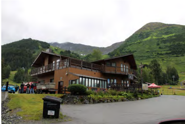
Figure 177. 210 Arlberg Avenue, view to the east.
