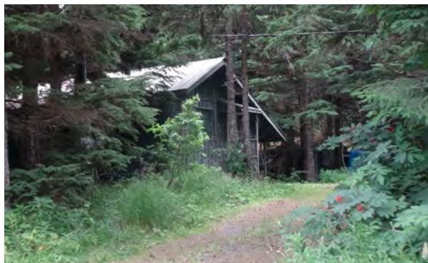
Figure 47. 142 Sproat Road, view to the northeast.
