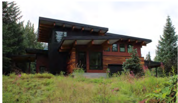
Figure 17. Decoupage style residence located in Girdwood, Alaska.
