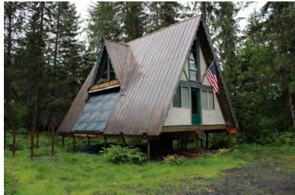
Figure 112. 139 Kitzbuhel Road, view to the south.
