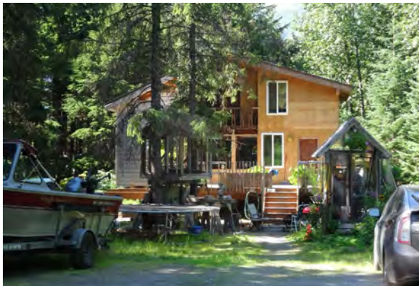
Figure 166. 207 Banff Circle, view to the west.
