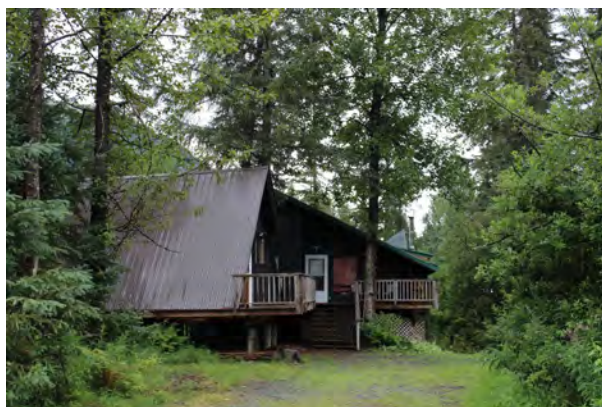
Figure 134. 275 Cortina Road, view to the south.
