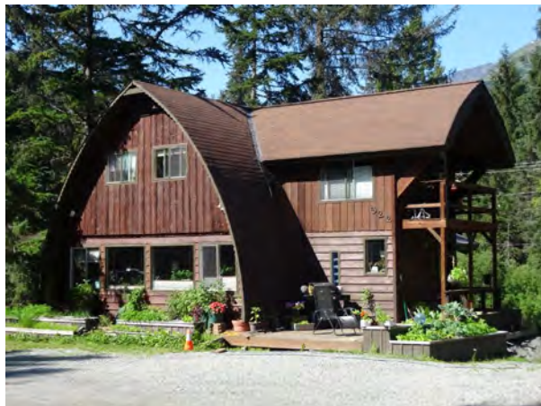
Figure 155. 322 Brighton Road, view to the northwest.
