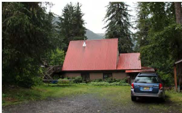
Figure 107. 257 Garmisch Road, view to the south.
