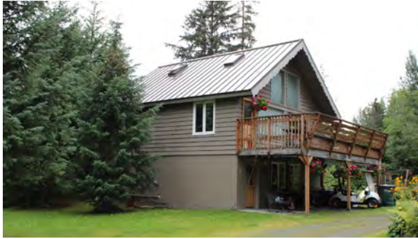
Figure 136. 128 Davos Road, view to the north.
