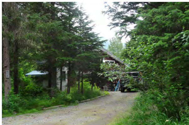
Figure 50. 616 Sproat Road, view to the northeast.
