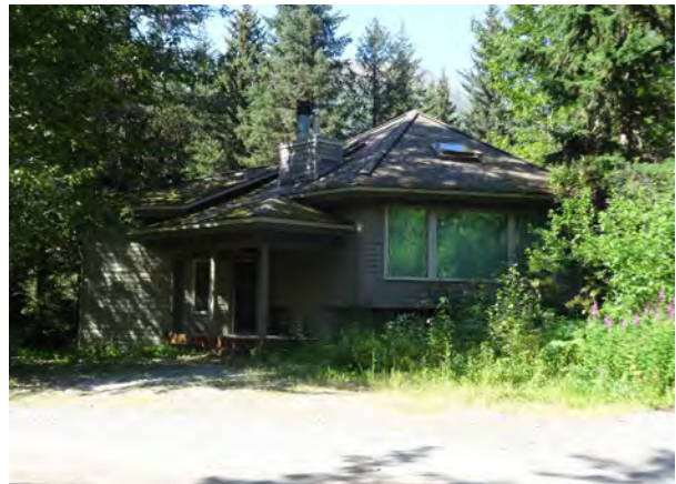
Figure 164. 243 Donner Drive, view to the west.
