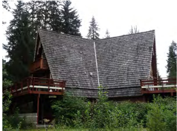
Figure 185. 663 Alyeska View Avenue is an unusual configuration of three separate A-Frame structures. The uniqueness of the structure could qualify it for eligibility under Criteria C.
