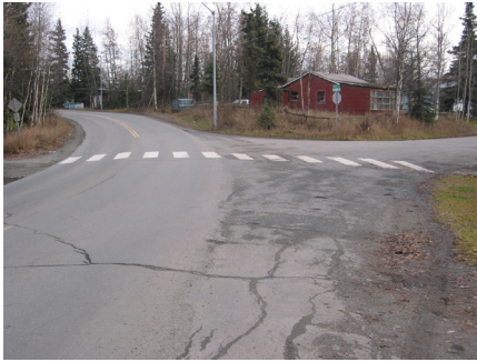
Before: 35th Avenue and McRae Road was a typical strip-paved “Spensard Street” with limited right-of-way and on-street parking. (photo courtesy of CRW Engineering Group)
