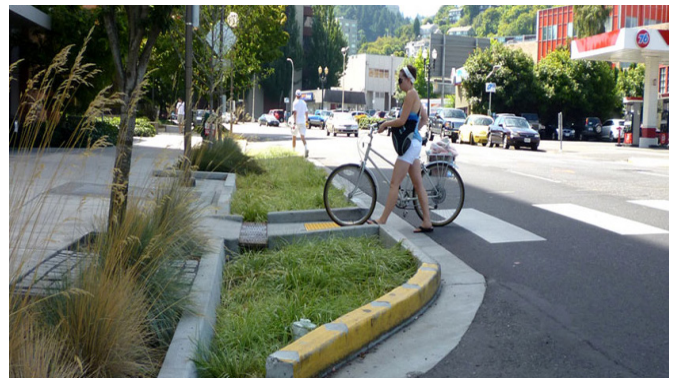
At-grade mid-block crossing
