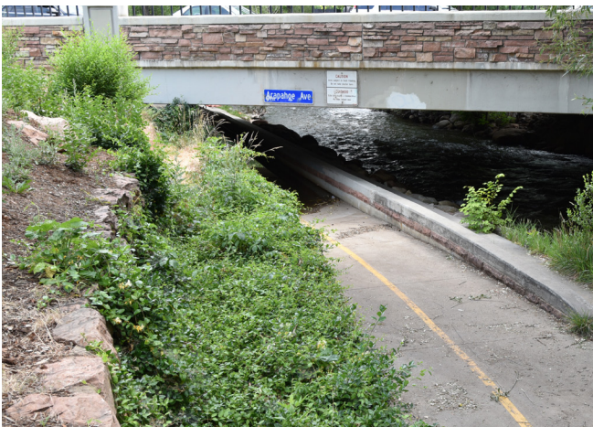
Grade separated crossing (undercrossing)
