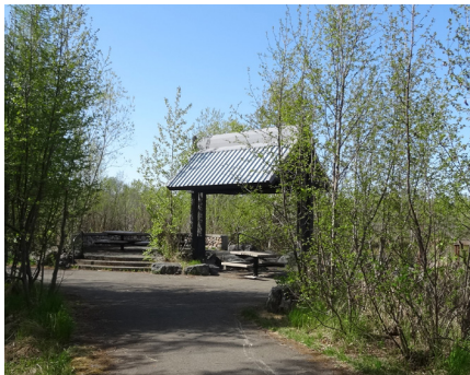
Encourage private development to provide public access to natural features, such as Fish Creek.
