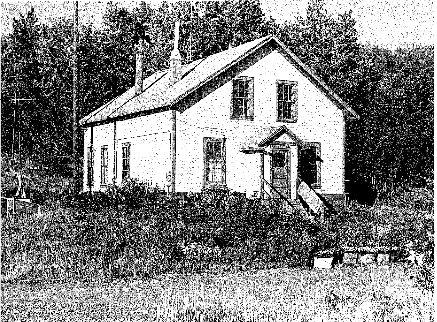
Potter Section House. Built by the Alaska Railroad in 1929, this section house is the only one of its type remaining along the rail belt.
