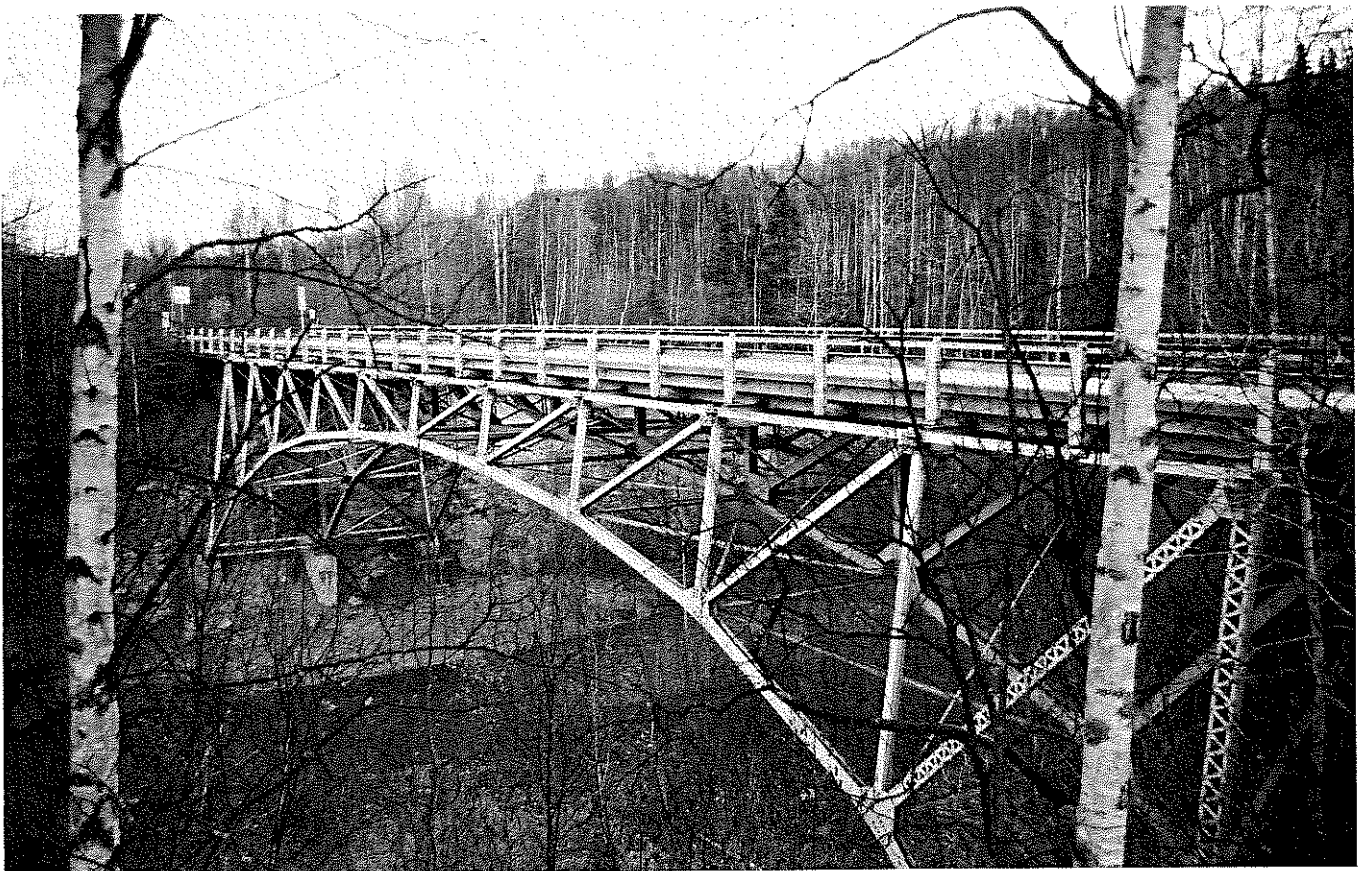
Eklutna River Bridge.
