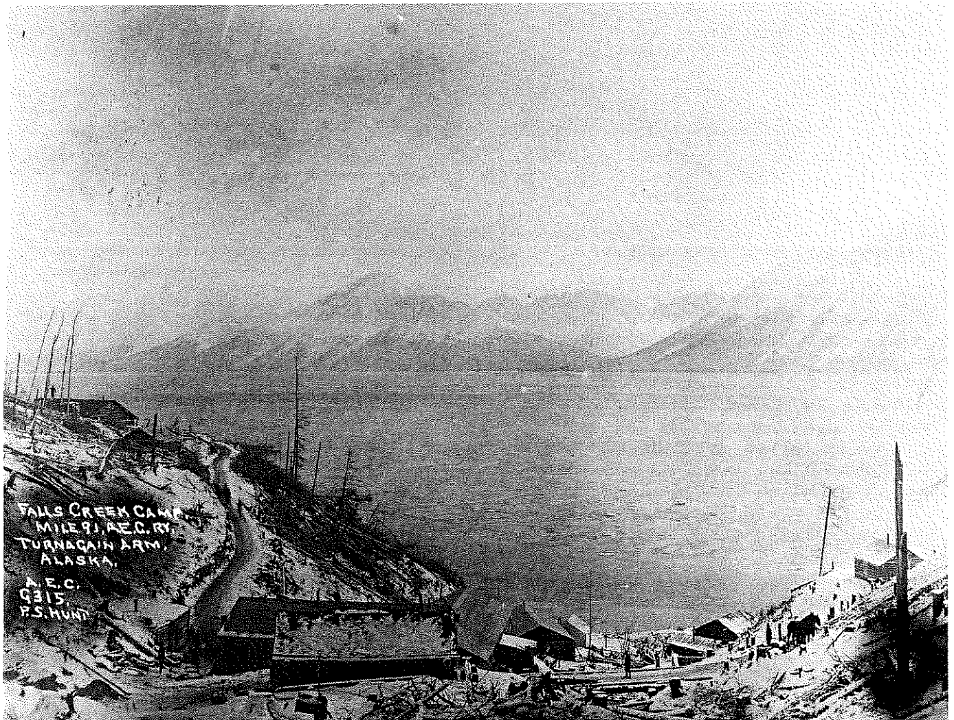
Falls Creek, 1917. Note the construction road - "the Johnson Trail" - heading down the Arm.
