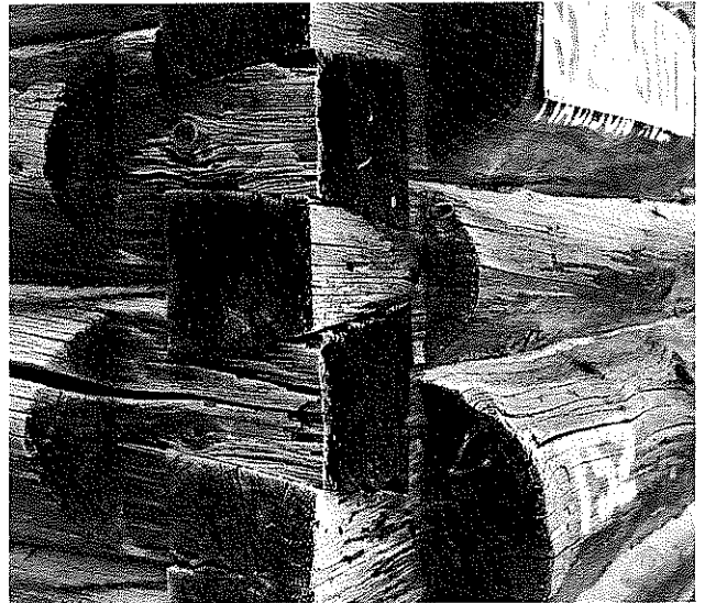
Dovetailed notching on round logs.
