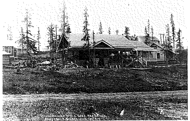
Commissioner Edes House as it appeared during construction in June 1917.
