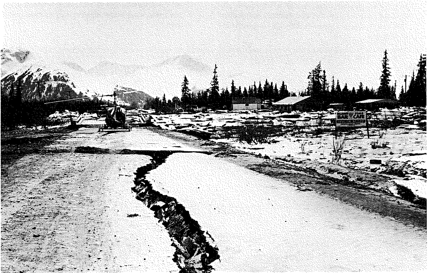
Portage 1964. After the Earthquake, the town was described as "almost a total loss." As the Seward Highway bridges were destroyed, it could be reached only by air.
