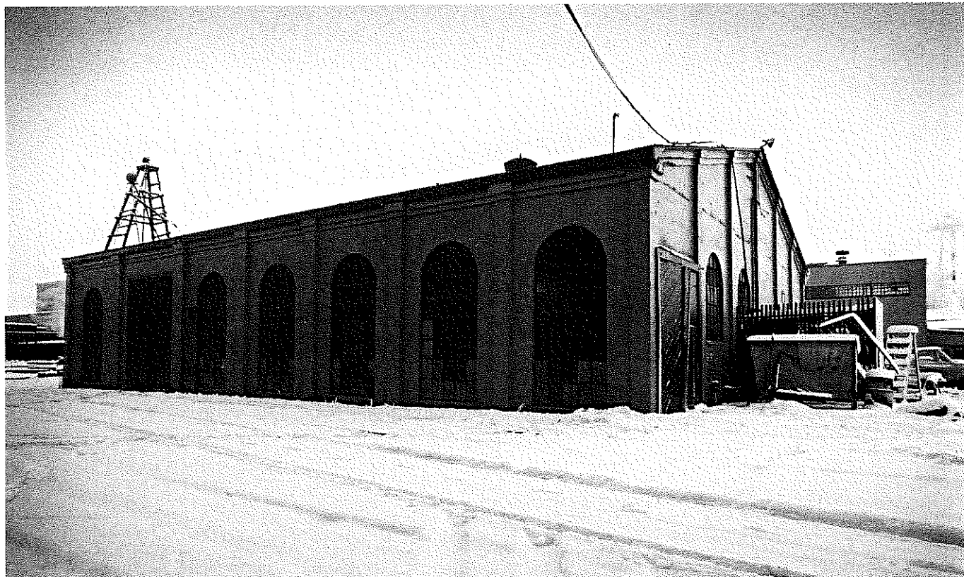
The Power Plant. Built by the A.E.C. in the early 1920's, it served both the railroad and Anchorage until the completion of the Eklutna Power Plant (1929).
