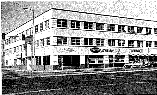
Loussac-Sogn Building today.
