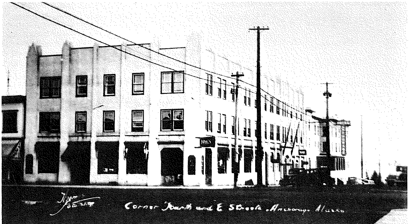
The Anchorage Hotel Annex in the 1940s.
