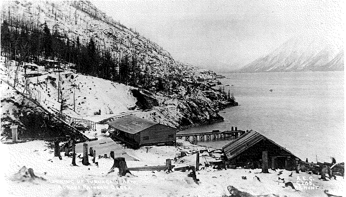
Construction camp at Rainbow Creek.
