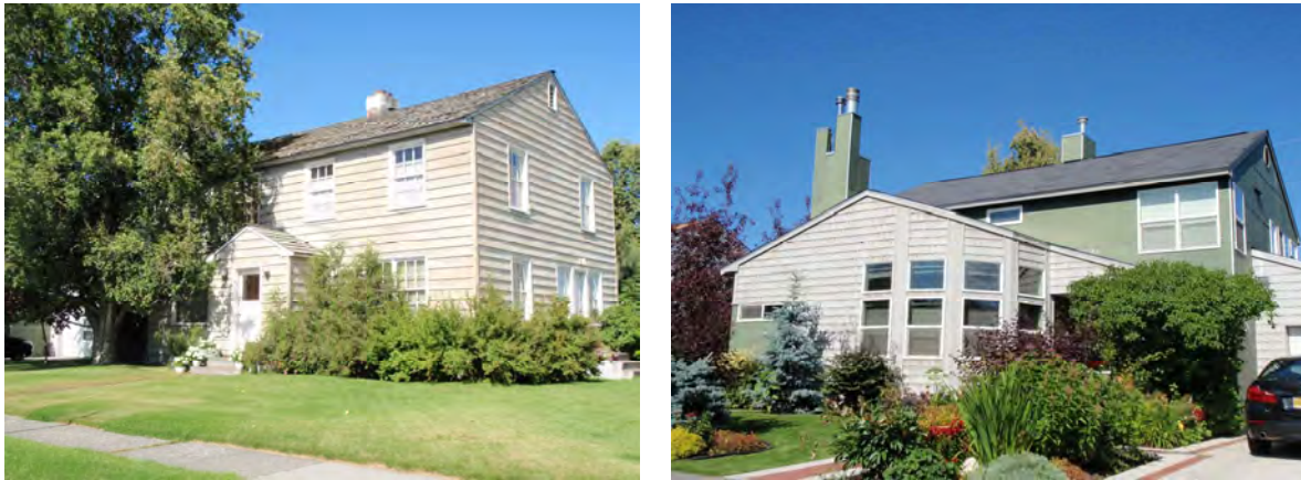
Pair of houses, originally of identical design and construction. The house on the left has had a few minor alterations but retains sufficient integrity, while the form, massing, and cladding of the house on the right have all been dramatically altered.
