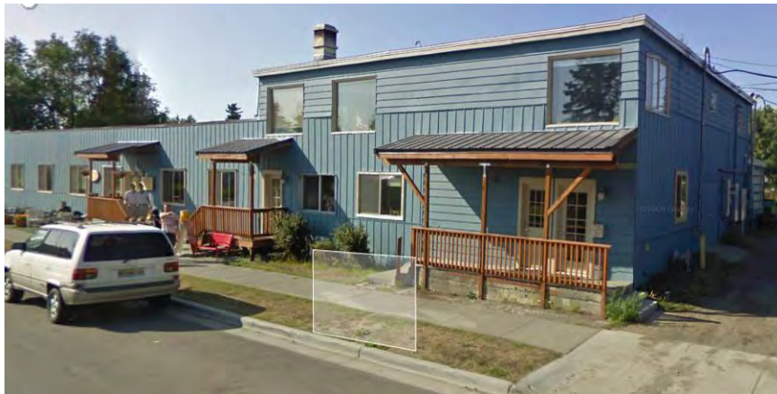
Mixed-use; residence over a shop (Photo from Google Maps, 2011)
