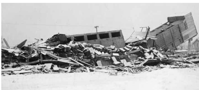
Figure 66. Four Seasons Apartments, 1964, following the Good Friday Earthquake. (Alaska Digital Archives, #UAF-1972-153-9)
