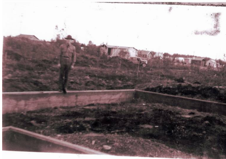
Figure 33. Lt. Bert Perrin at the foundation of his future house on Block 13. (Courtesy M & M San Angelo)
