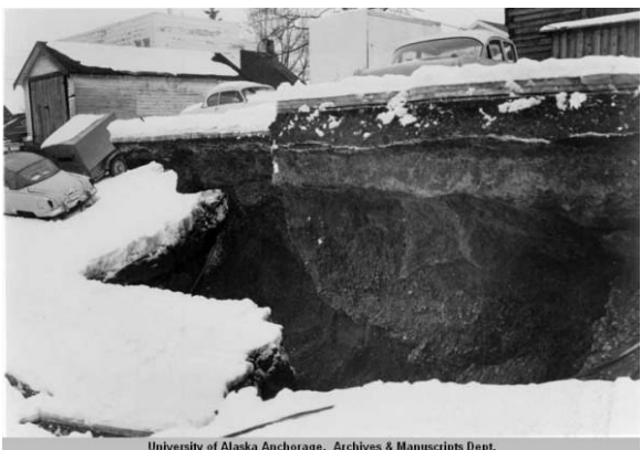
Figure 64. Earthquake damage along L or N Street, 1964. (Alaska Digital Archives, #UAA-hmc-0427-10)
