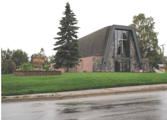
Anchorage Lutheran Church, 1420 N Street
