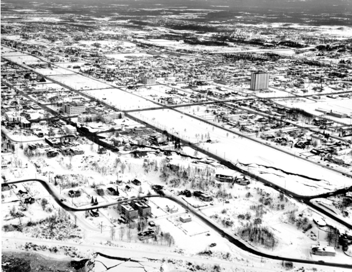
Figure 62. Aerial view of the Park Strip and South Addition, showing earthquake damage along the L Street Slide in the foreground (1964). (Army Corps of Engineers 1964 Earthquake Photographs Collection; Anchorage Museum #B1977.118.96)
