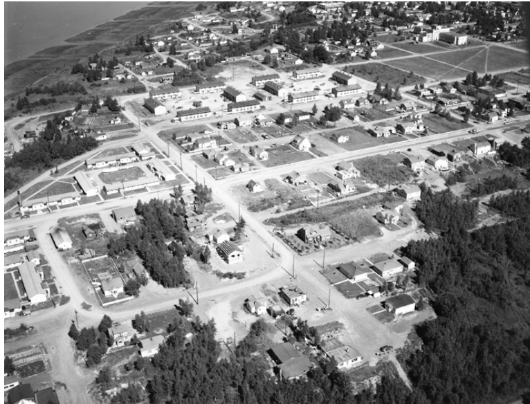
Figure 39. Aerial view of 11 th Avenue and P Street after the war, 1948. This photo clearly shows the World War II barracks at the west end of the Park Strip (between N and P streets), Safehaven, scattered residential development, and a handful of small vegetable gardens. (Steve McCutcheon, McCutcheon Collection; Anchorage Museum, #B1990.014.5.AncAir.5.1.30)
