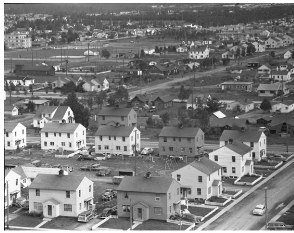
Figure 38. Detailed view of CAA duplexes at 13 th Avenue and I Street from roof of 1200 L Street, 1951. (Steve McCutcheon, McCutcheon Collection; Anchorage Museum, #B1990.014.5.AncAir.3.13)
