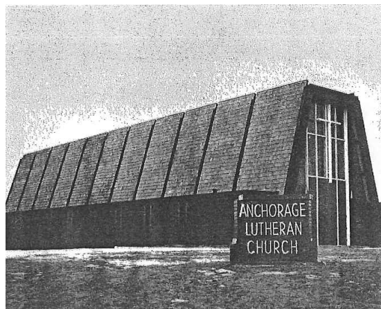
Figure 60. Anchorage Lutheran Church, 1960s (Chamber of Commerce Brochure, in Anchorage Museum Vertical Files)
