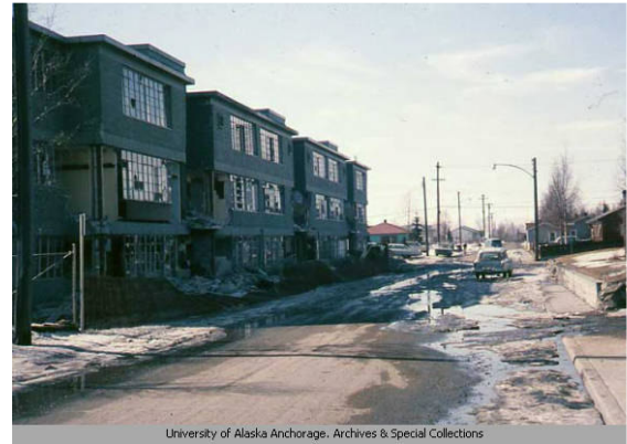
University of Alaska Anchorage. Archives & Special Collections Figure 48. Hillside Apartments in 1964, after Good Friday Earthquake. (Alaska Digital Archive, #UAA-hmc-0809)
