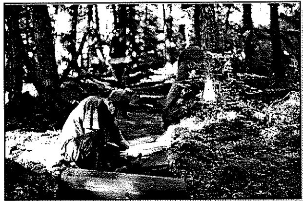
Student Conservation Association crewmember installing geotextile material on Upper Glacier Creek segment of proposed Iditarod Trail.
