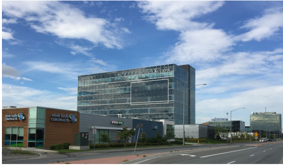
Buildings Oriented to 36th Avenue in Midtown
