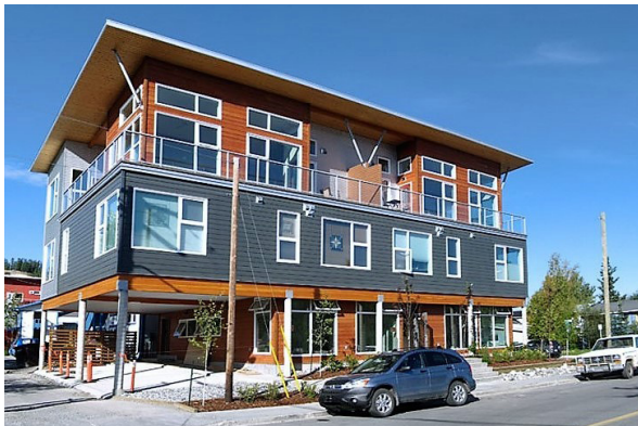
Residential Mixed-use in Whitehorse. Ground-floor Commercial Contributes to Street Activity.
