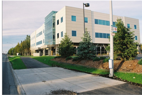
Street-facing Medical Services Building on Lake Otis Transit Route
