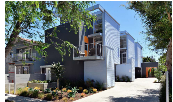
Small-lot Single-family Homes, Each on its Own Lot. Shared Driveway and Utility Easements. Front Unit is Oriented to the Street with Front Entrance and Path.
