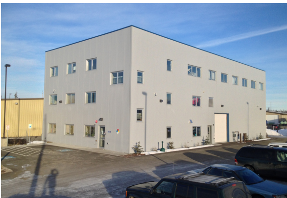
Office-Warehouse with Environmental Tech Services Firm
