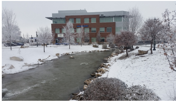
Indian Creek Daylighting and Urban Revitalization in Downtown Caldwell, ID
