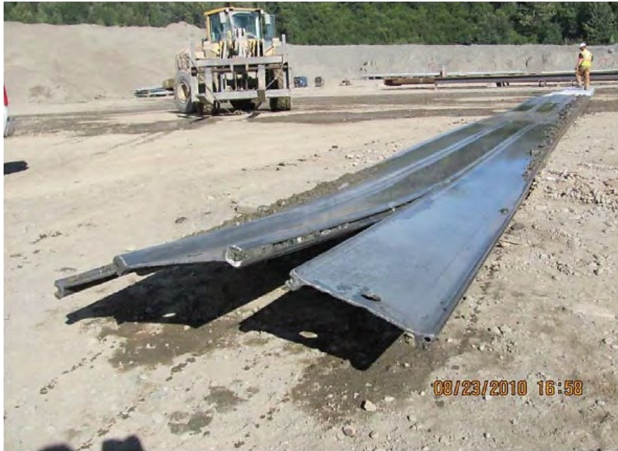
Sheet pile “unzipping”
