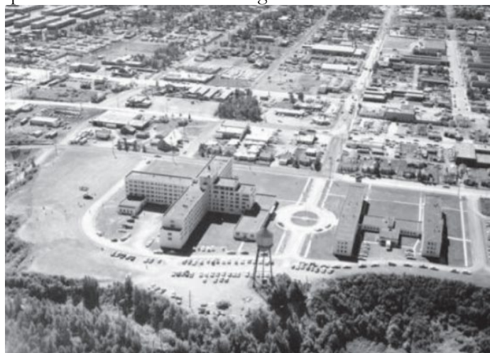
Figure 1 Former Alaska Native Service Hospital, 1960
