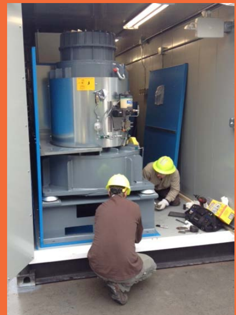
Figure 22. Installing ABB Flywheel in Kodiak Photo: Courtesy Darron Scott
