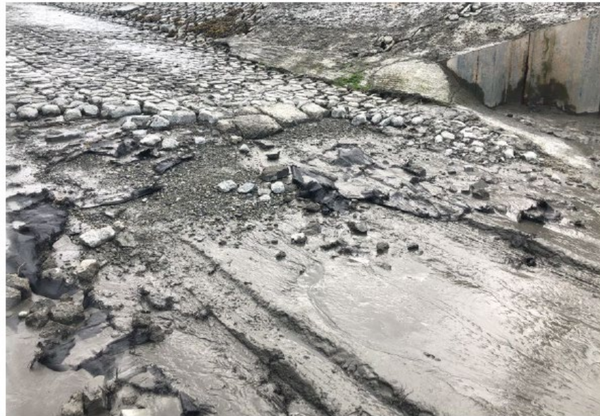
Photo 10: 2021 Project – South Ramp Repair Area (2020)
