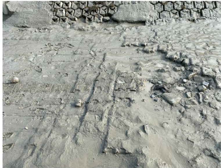
Photo 8: North Ramp -ACB circa 1987 (right) and ACB Repair circa 2008 (left) (2020)
