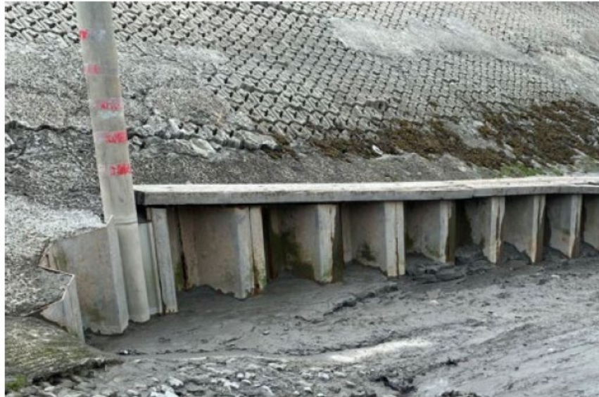
Photo 12: 2021 2021 Project – South Backslope Repair Area (2020)
