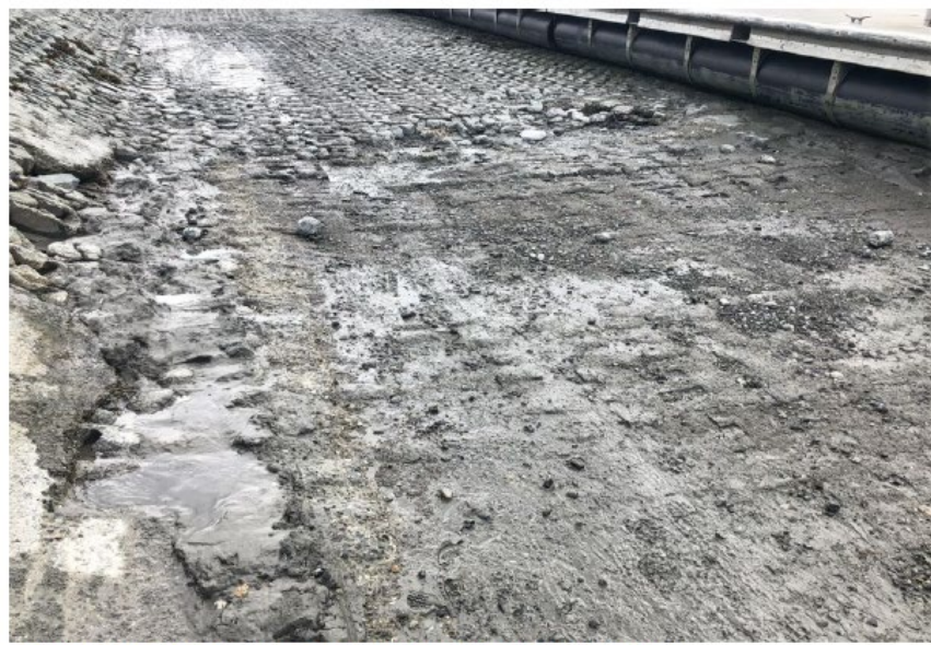
Photo 11: 2021 Project – North Ramp Repair Area (2020)
