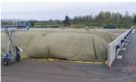
Photo 3.3: Membrane Covered Aerated Static Pile
