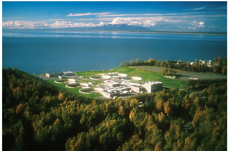
Photo 4.1: Asplund Waste Water Treatment Plant
