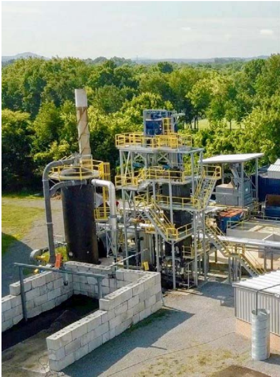
Figure 2-3: Gasification Plant in Lebanon, Tennessee (64 tpd, 1.8M kWh)
