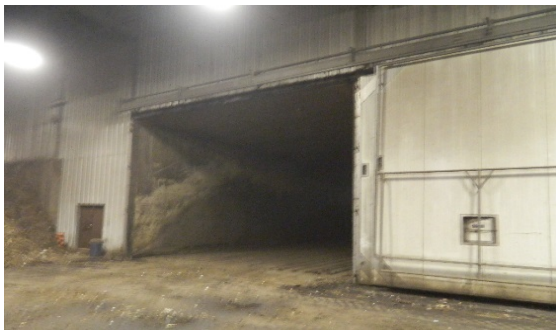
Photo 3.4: In-Vessel Composting Bunker
